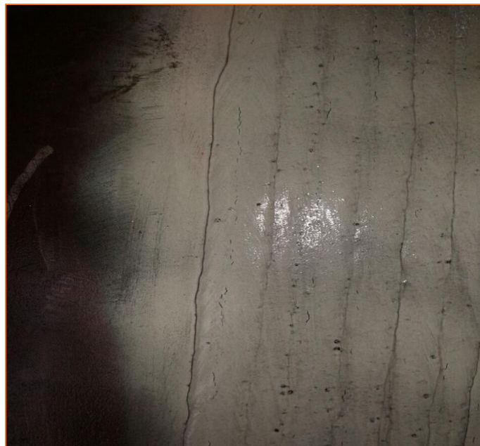
Fig 1: Cracks appeared throughout the SAW weld
