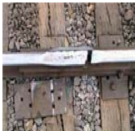
Figure 5: Detection of cracks.
