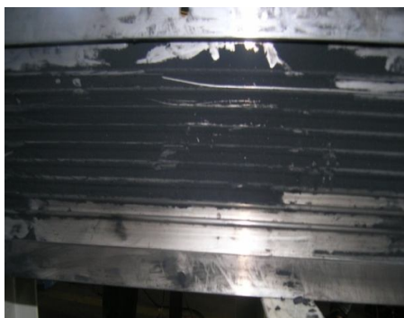
Fig. 7: Busduct after Fire Survival Test
