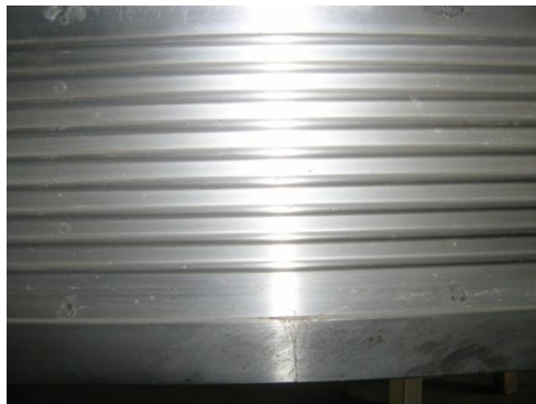
Fig. 5: Busduct before Fire Survival test
