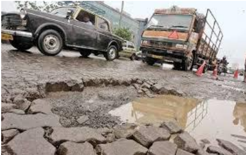
Figure 2. Spilling over of sewage on the road
