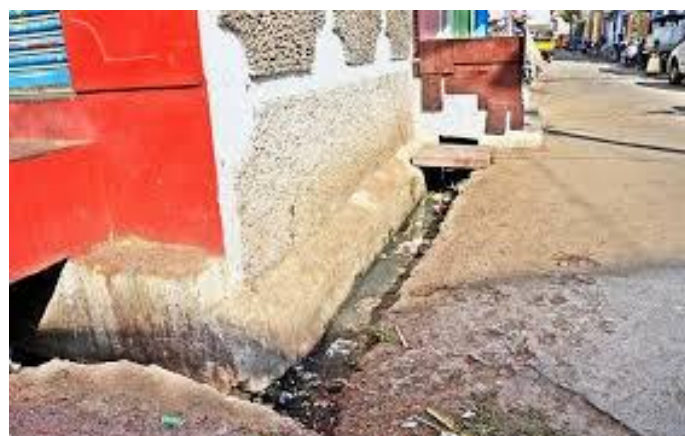
Figure 5. Drains on the Road
