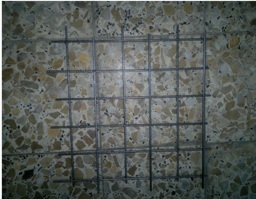
Fig 4 Deformed bars reinforcement
