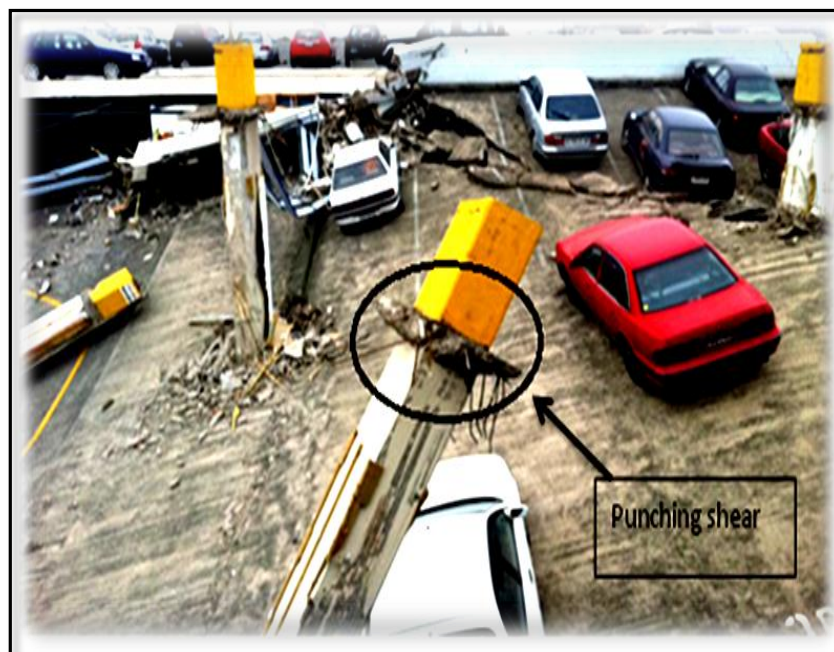
Fig 2 Punching shear failure
