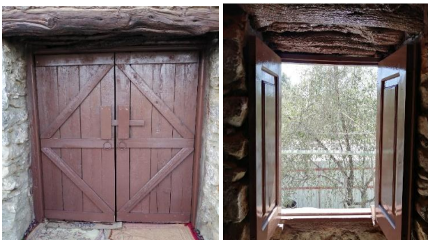
Fig. 19. The new door and window
