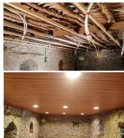
Fig. 16. Roof before and After Refurbishment
