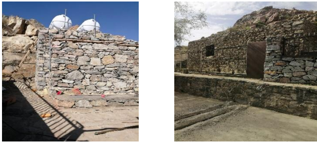
Fig. 17. The new construction surrounding wall, bathrooms and flagstones
