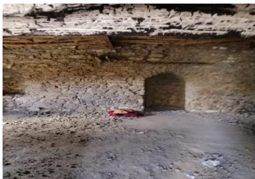
Fig. 15. Abrade wall during the refurbishment
