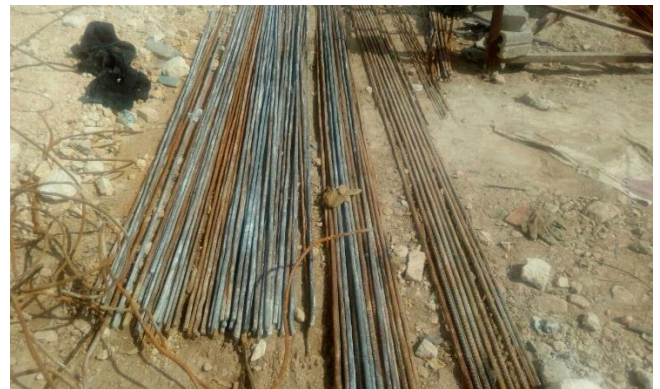
Figure 5. Sorting of steel bars
