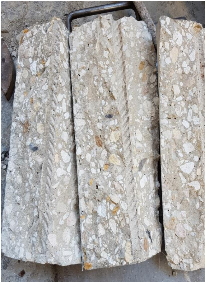
Figure 8. Fresh indentations of deformed steel bar after division
