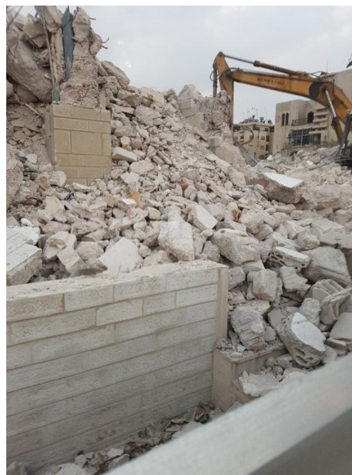
Figure 1. A location for demolition in Amman
