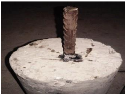
Figure 9a: Pull through failure mode
