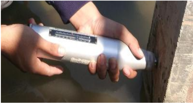
Fig 3. Rebound Hammer Test Equipment
