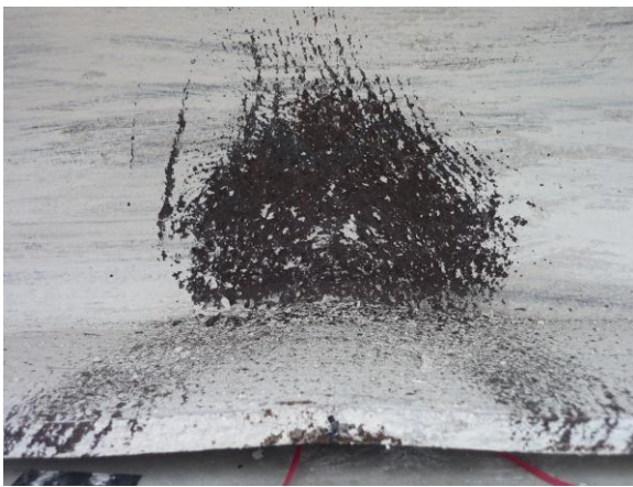
Figure 10. Steel beam failure SCCB-S1-SM-01.
