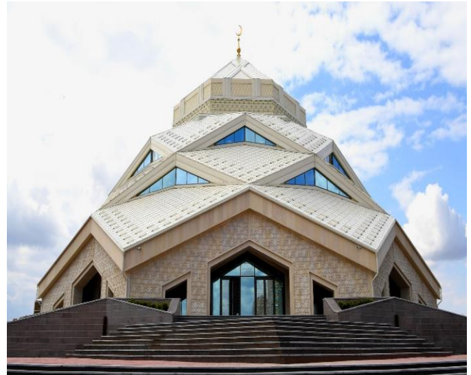
Fig. 8. A general view of the Yrskeldy Kazhy Mosque in Nur-Sultan
