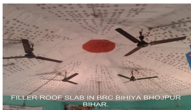
Fig.5: The use of filler slab in study area Block Resources Centre, Bihiya
