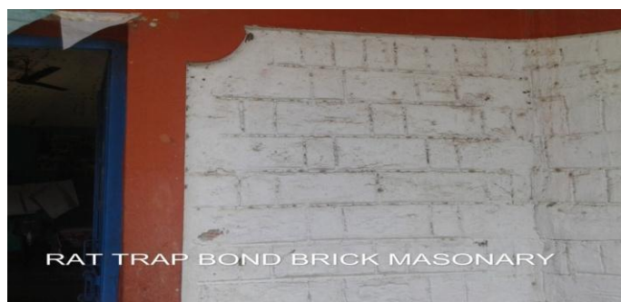
Fig. 4: Rat Trap Bond masonry of Block Resources Centre, Bihiya District-Bhojpur, Bihar
