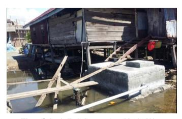
Figure 5. Septic Tank Construction of Study Object
