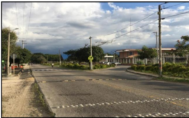
Fig. 2. Eastbound access road.
