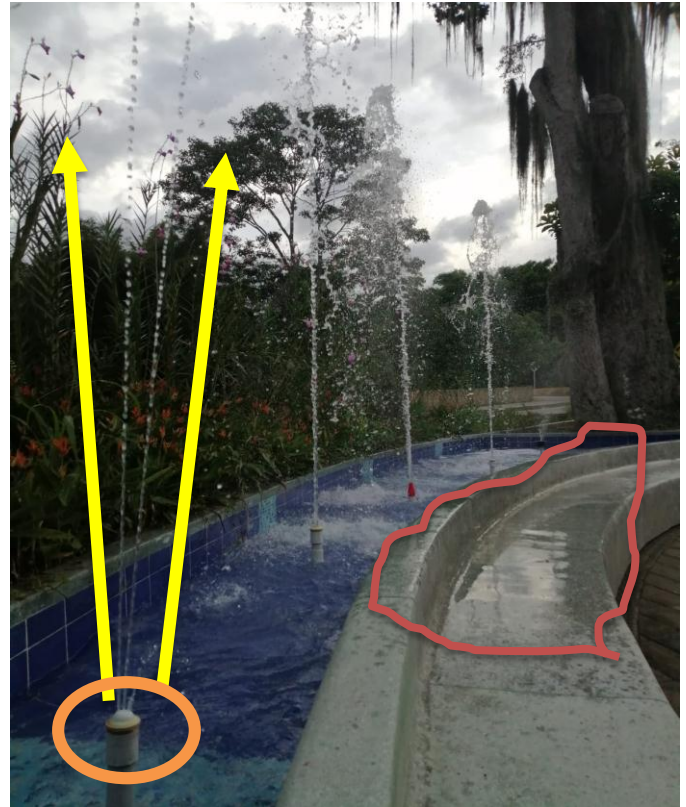
Fig. 2. Problems caused by malfunctioning nozzles.
