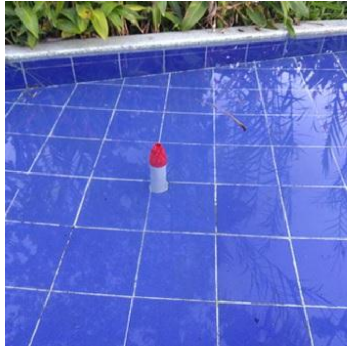
Fig. 11. Installed and functional part.
