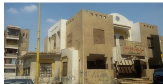
Fig. 3. The Motherhood and childhood care center building from the main front façade
