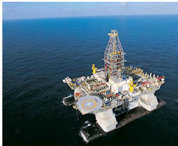
Figure 1b: Deepwater Horizon semisubmersible rig[1]
