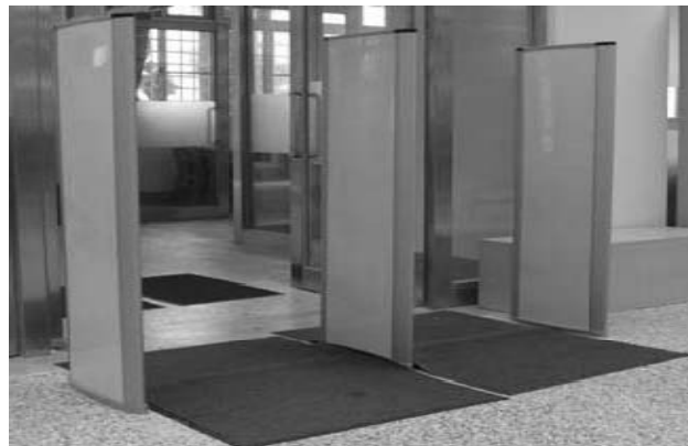
Figure 5: Exit sensors (Double Aisle)
